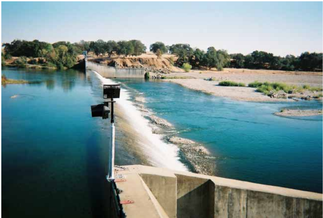
Figure II-a. Daguerre Point Dam (photo by D. Simodynes, October 9, 2009).
