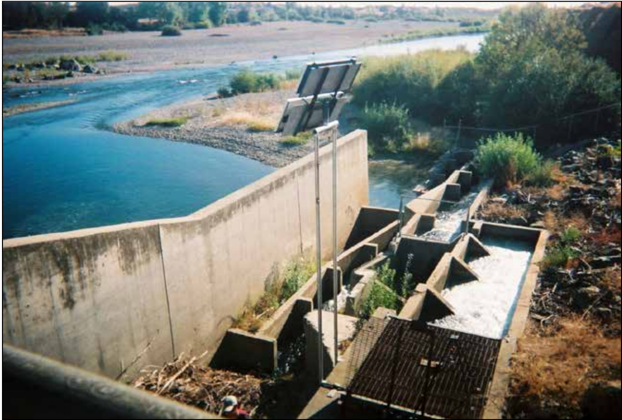
Figure II-b. North fish ladders at Daguerre Point Dam (photo by D. Simodynes, October 9, 2009).
