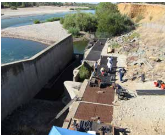
Figure V-a. Installation of metal grates on the Daguerre Point Dam fish ladder bays during August 2011 (from biological assessment).
