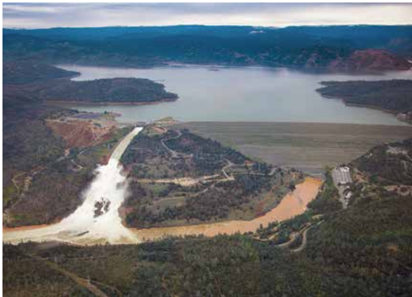
Oroville Dam's Main Spillway at 100,000 cfs. An aerial view looking eastward toward Oroville Dam and Reservoir. The emergency spillway is on the left (note eroded red dirt area) and the damaged main spillway left of center. Oroville Dam is on the right. An outflow of 100,000 cfs travelled down the main spillway on Feb. 15, 2017. Source: Dale Kolke, DWR.
