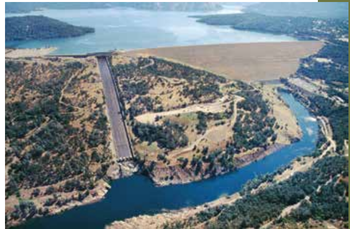
Oroville Dam. This aerial photograph was taken before 2017 and shows the dam on the right side, the concrete main spillway in the middle, and the emergency spillway on the left with a vegetated hillside below. Source: DWR.
