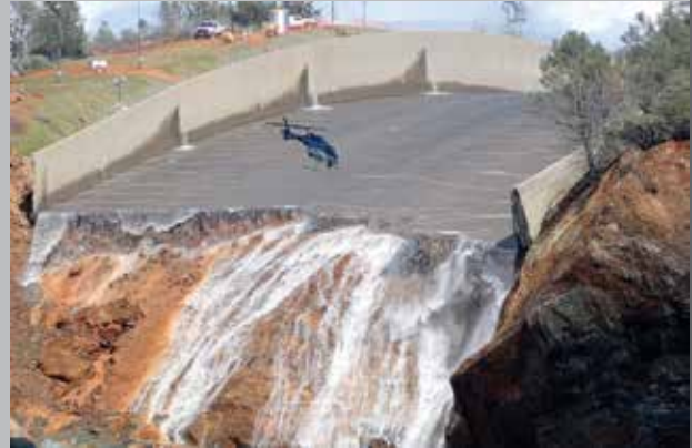
Main Spillway, Feb. 27, 2017. As DWR decreases flows on the damaged main spillway to assess damages. Source: Bill Husa, Chico Enterprise-Record.
