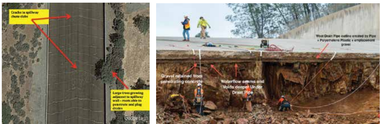
Oroville Forensics. Bea points out the many cracks on the surface of the spillway, as well as trees growing too close to the edge of the structure in this 2010 satellite image (left). Bea believes a hidden drain pipe proved the critical weakness along the spillway (right). Image source: Bea, Root Causes Analysis, using GoogleEarthPro and DWR images.
