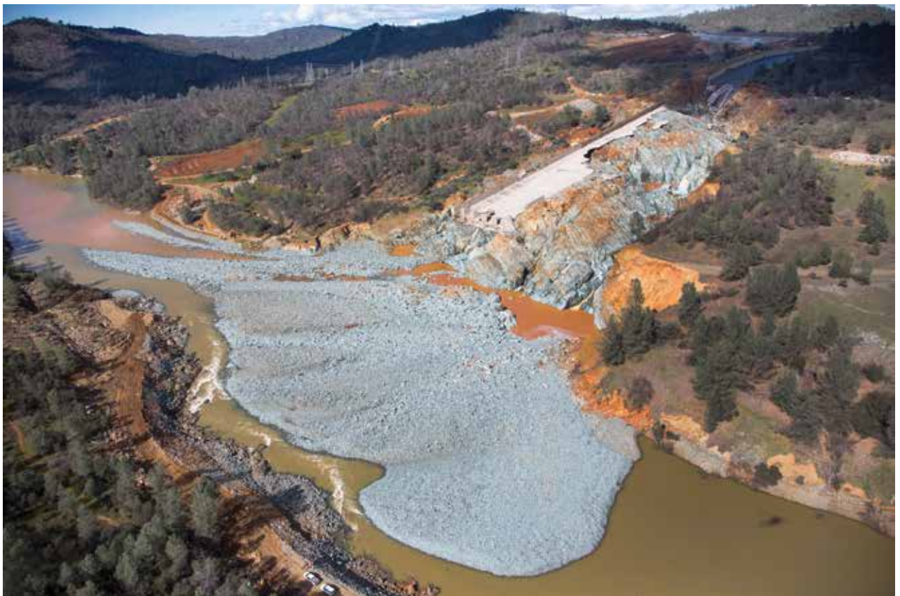
Damaged Main Spillway, Feb. 27, 2017. An aerial view of the damaged main spillway and resulting debris field. Flows were reduced from 50,000 cfs to zero on Feb. 27 to allow reduction of the water elevation in the diversion pool, removal of debris, and re-initiation of power generation at the Edward Hyatt powerhouse. Source: Dale Kolke, DWR.
