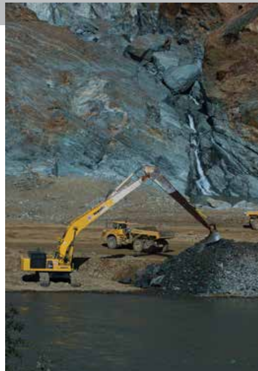
Removal of debris from Feather River diversion pool. Source: DWR
